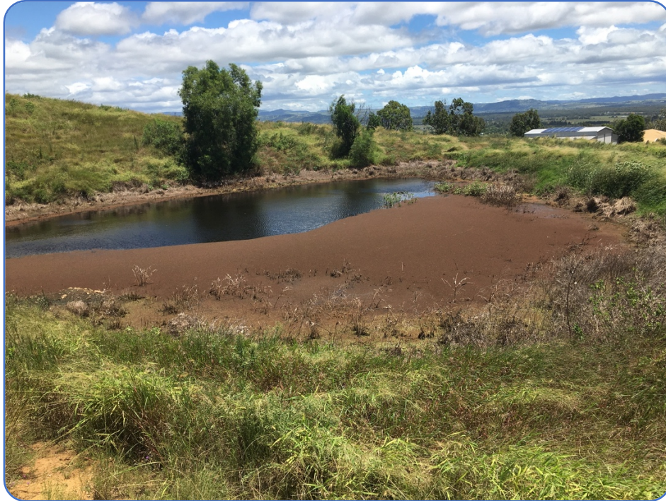
Figure 6.4 Dam located in the central west
