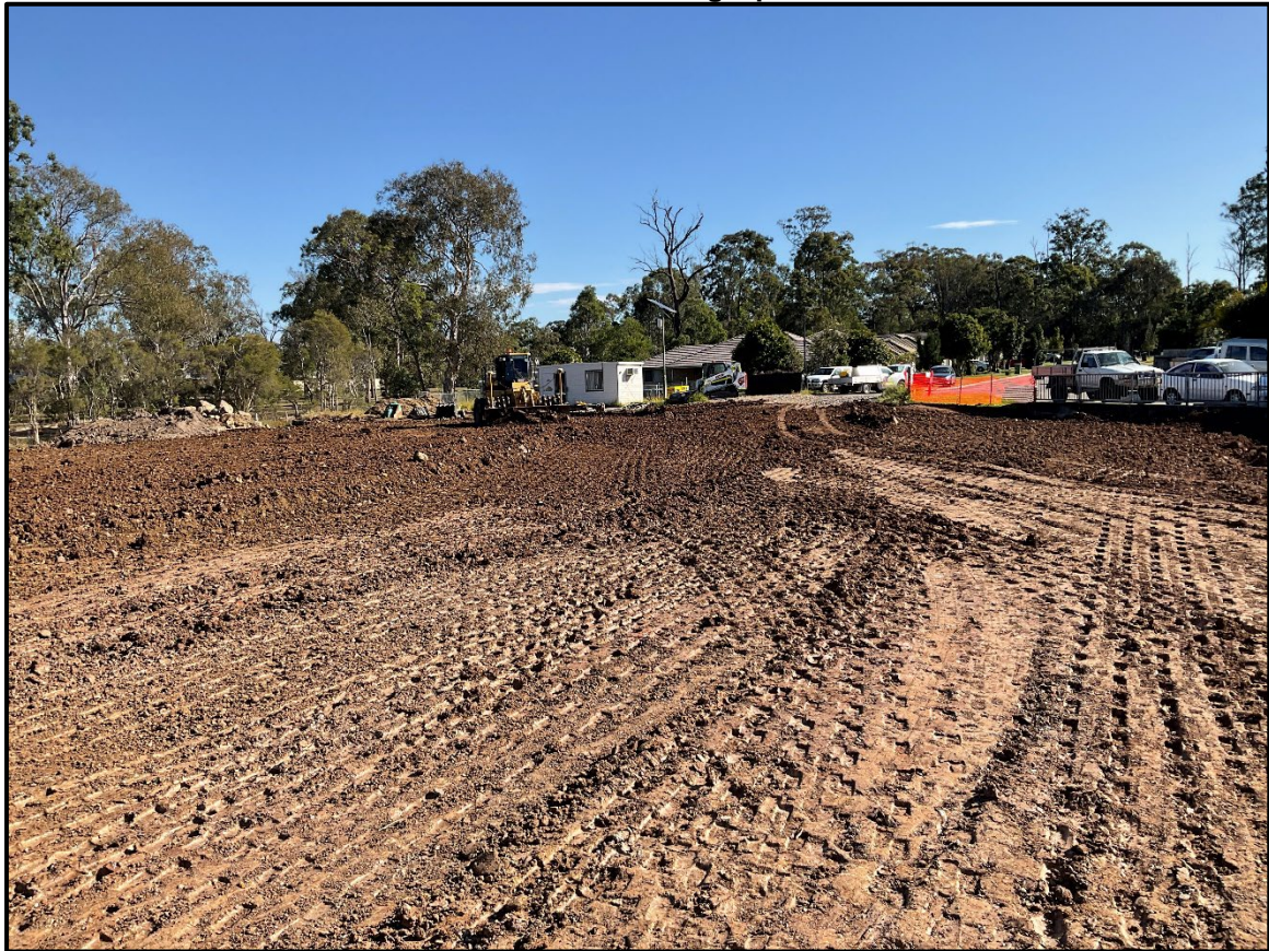
Picture 2: View of Filling Operations
