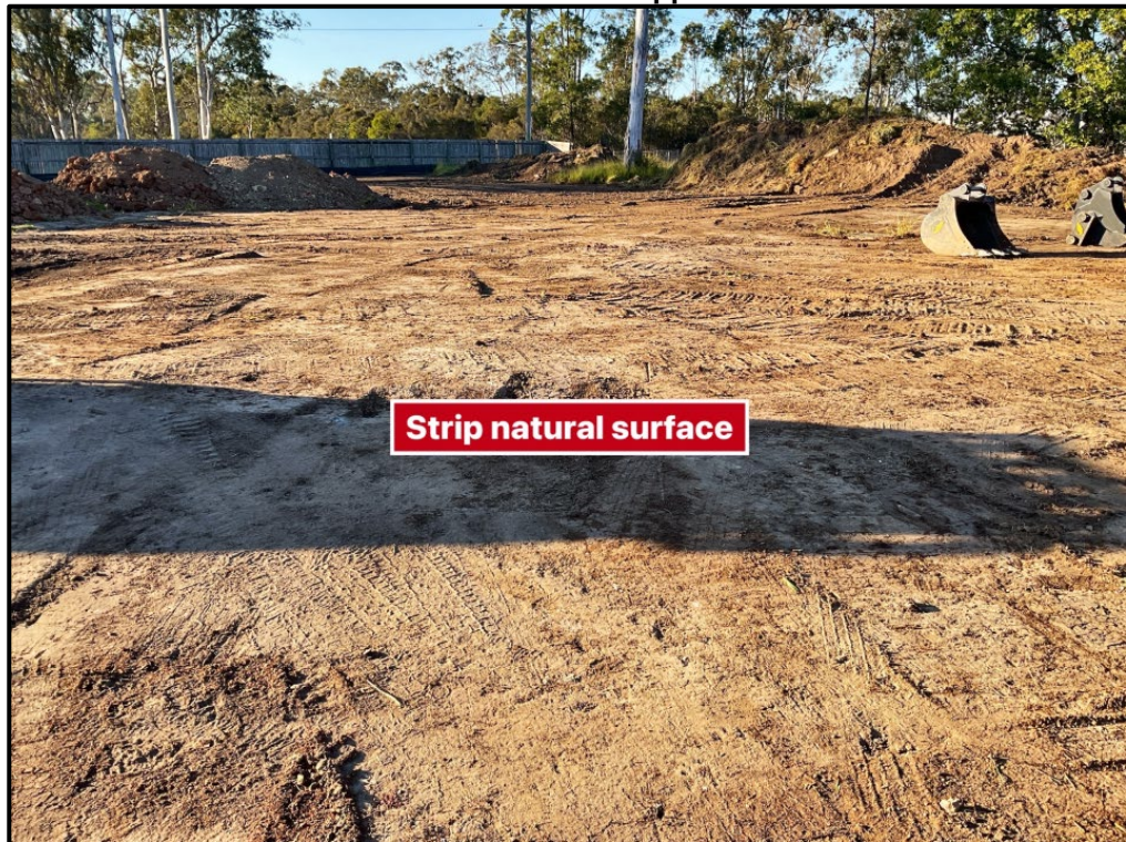
Picture 1: View of the Stripped Surface
